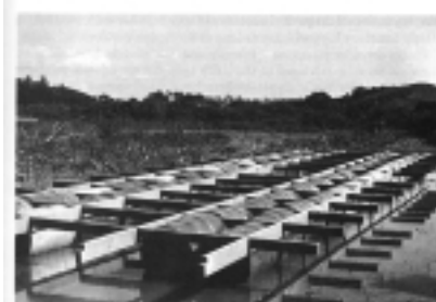
Figure 2-6. Barrels beneath a raft frame support the 54-foot houseboat shown in Figure 2-7.
